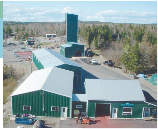
Aerial view of the Future Nets facility showing net loft, storage areas, cage manufacturing plant and the newest addition, an 82-foot high net drying tower (right).
